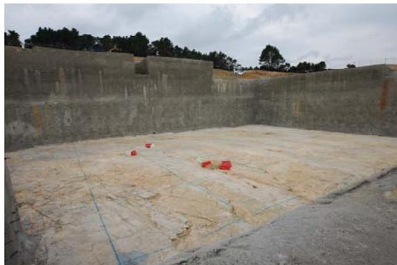
The floor of the future nuclear reactor unit, dug into the rock (300000m<sup>3</sup> removed).
